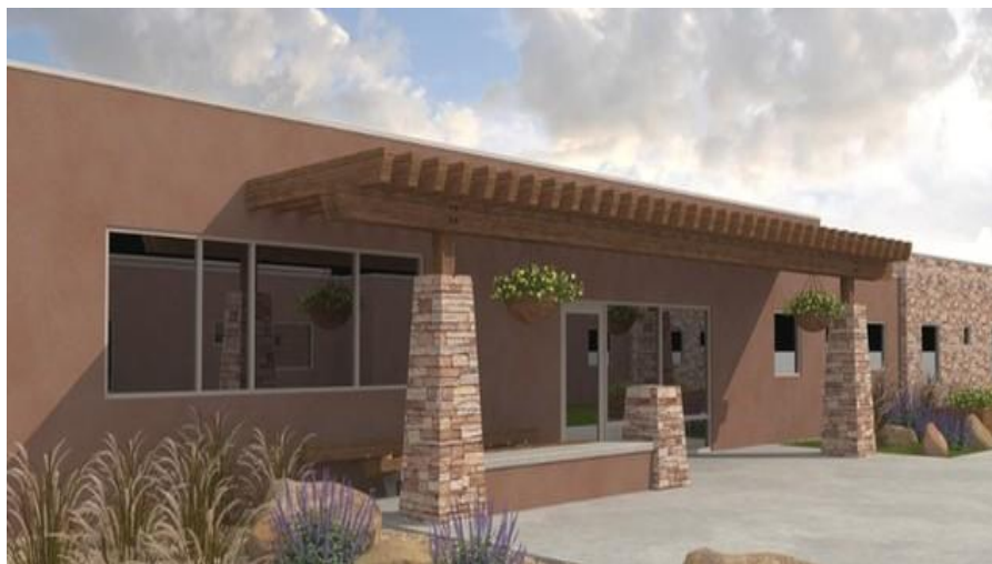
An artist's rendering shows how the new 108-bed Utah State Veterans Home in Ivins will look when completed
